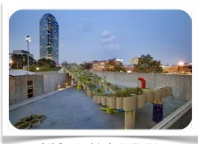
Public Farm 1 Installation, Brooklyn, New York Source: Public Farm 1
