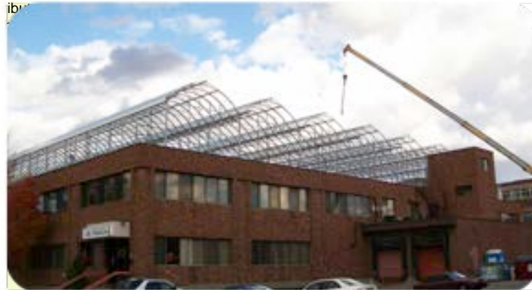
The Construction of Lufa's Rooftop Greenhouse Source: Greenhouses Canada
